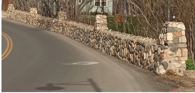
Stone and Mortar Wall. Old Town Cottonwood.
